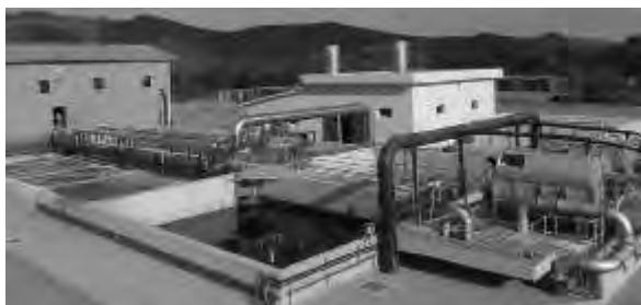
Figure 7: Ujams, Wastewater treatment, Water Reuse, Windhoek, Namibia (applying both MARAPUR and MICROPUR was started up during end of 2014 (5175 m 3 /d, DBOO contract)
