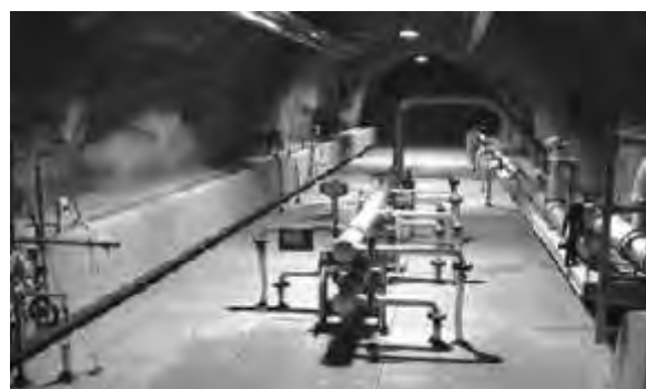
Figure 6: Swiss ski Resort Zermatt off-course no one wants to hear or see the WWTP so this plant finished by WABAG this year had to be placed under ground in a cave as well (12000 m 3 /d DB project).
