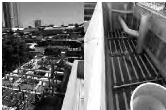
Figure 3: Nitrification basin with sieves installed ready to receive the FLUOPUR carriers.
